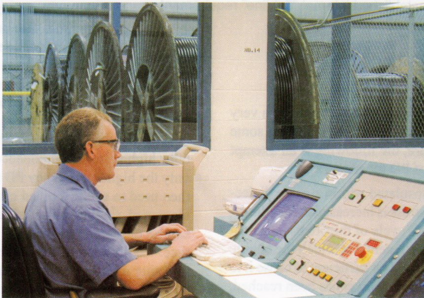
Corona Test is performed on a single conductor prior to cabling at Okonite's newly constructed Test Facility at our Orangeburg, SC Cable Plant.
